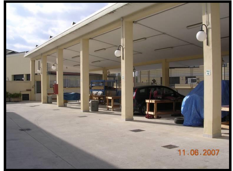
SS Hobby shop drainage
