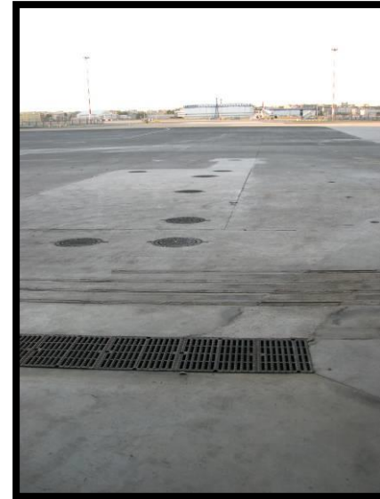
Capo Hangar 406 AFF collection Trench and Separator
