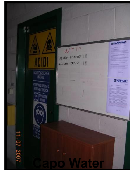
Capo Water Treatment Plant HM Storage
