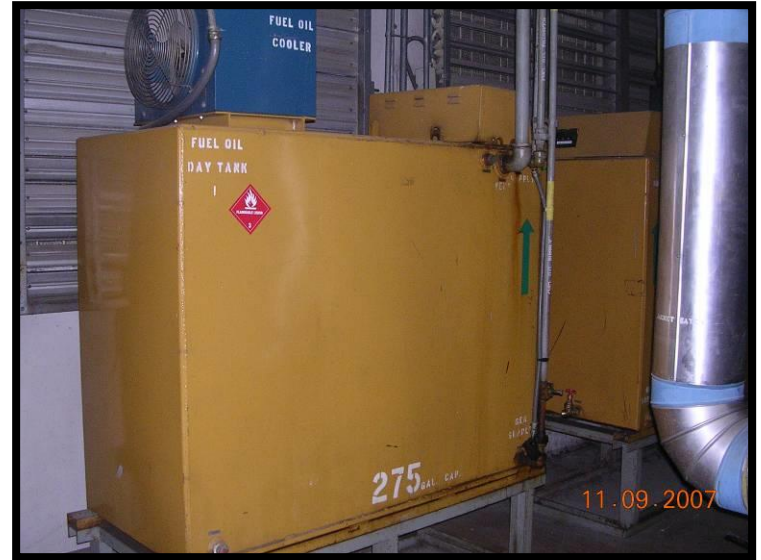
Capo C4I Generator Day tank
