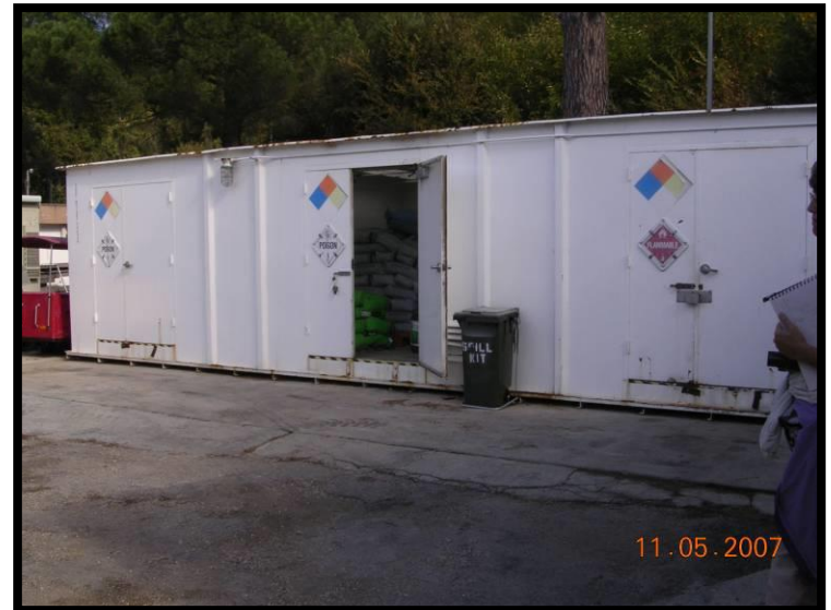
CP Building 516 HM Storage Lockers
