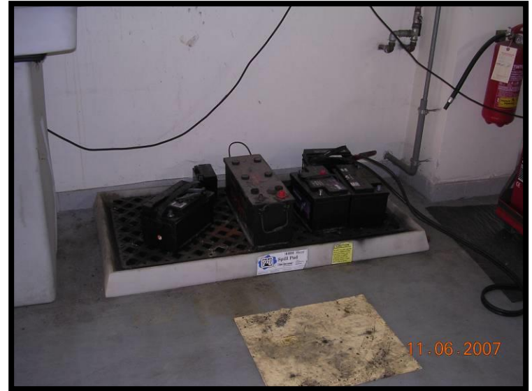
SS Hobby Shop Battery Storage
