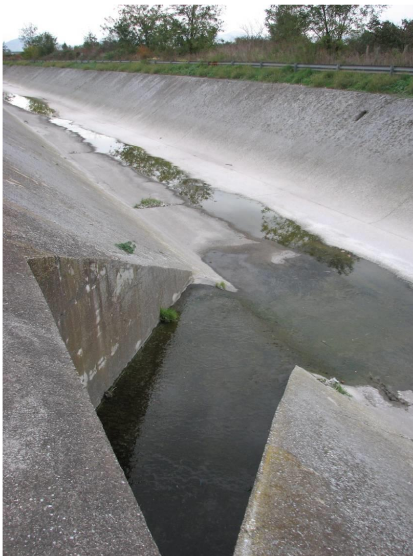
Figure 2-4 SS Gricignano Stormwater Outfall
