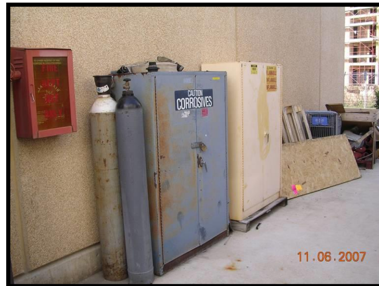
SS Hospital Generator Building HM Lockers
