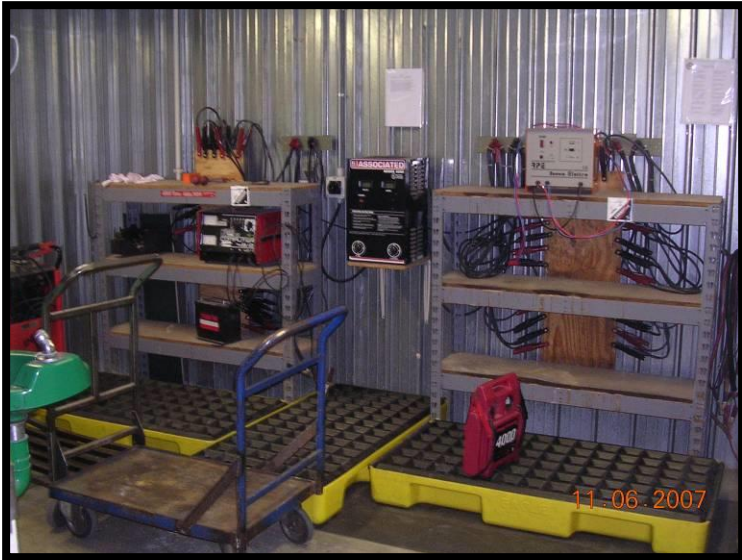
PW Transportation Battery Room
