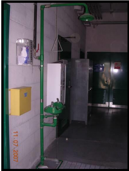
Capo Water Treatment Plant Eyewash/Shower
