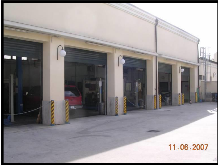
SS Hobby shop drainage 2
