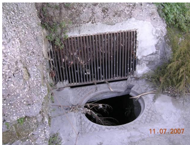
Figure 2-1 Capodichino Stormwater Outfall
