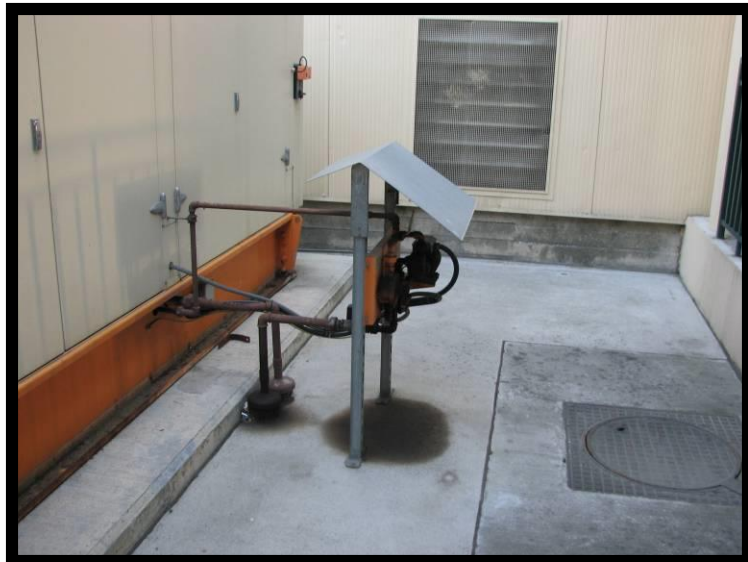
AST C-412 Piping to Generator
