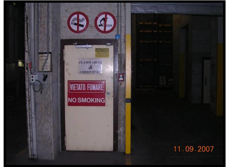
Capo Supply HM Storage BLDG 401
